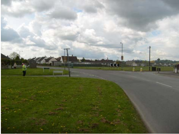
Exeter Road looking South
