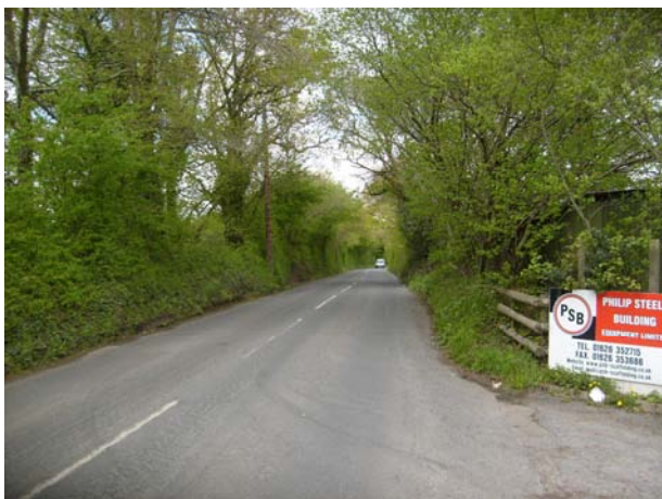
Broadway Road (North) looking West
