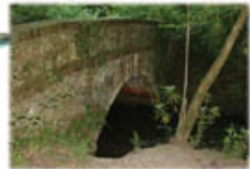
Bridge on carriage drive
