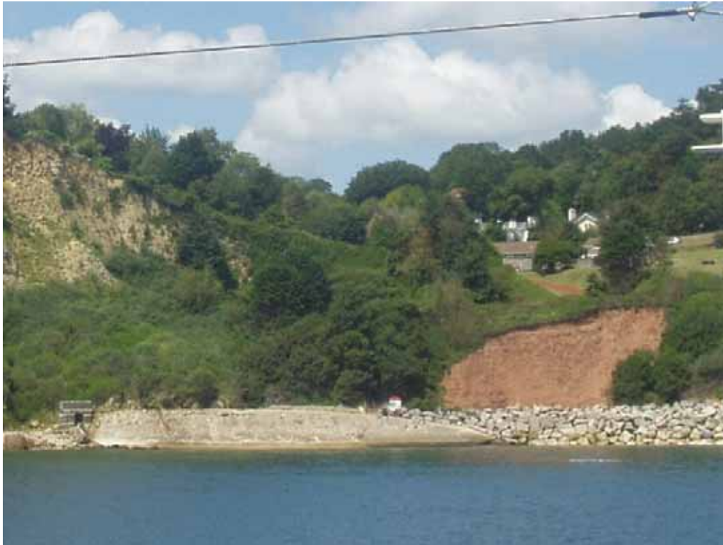
Seaton Hole viewed from the sea. Note Mercia Mudstone Group (Triassic) to the right downfaulted against Cretaceous to left. Platform represents coastal defence works
