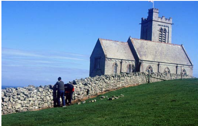
Lundy Granite used as a building stone on the island
