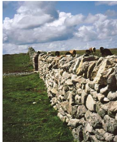
Rocks of Lundy Granite used to construct stone walls on the island
