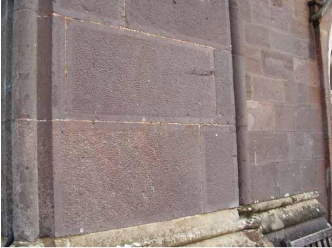
Killerton Chapel: built from lamprophyric Permian igneous rocks from the adjacent quarry.
