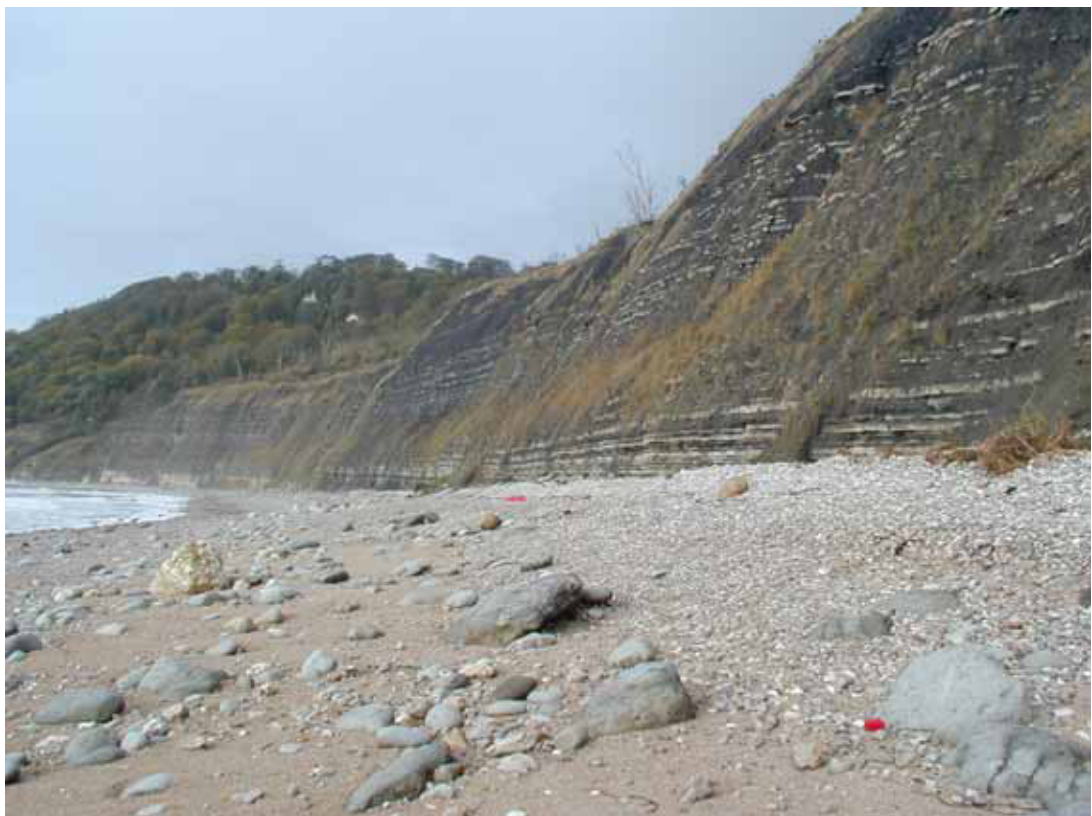
Two views of Pinhay Bay, the upper from the sea. Note the 'White Lias' (Lilstock Formation, Penarth Group- pale buff coloured limestones) – Blue Lias Formation (gray interbedded limestone bands and mudrock) boundary) near the base of the cliffs.
