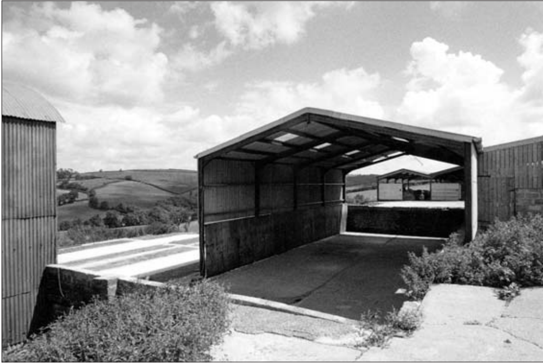
The empty silage clamp after it had been cleaned and disinfected
