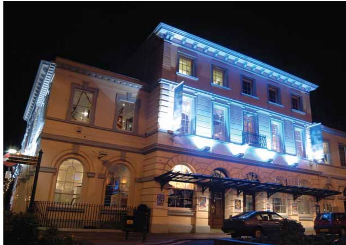
THE Queen's Theatre at Barnstaple (pictured above) has received £60,000 to replace five 25-year-old boilers with three new condensing boilers. The new boilers will save some
