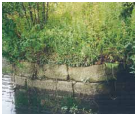
George Templer memorial stone, Jetty Marsh Lock
