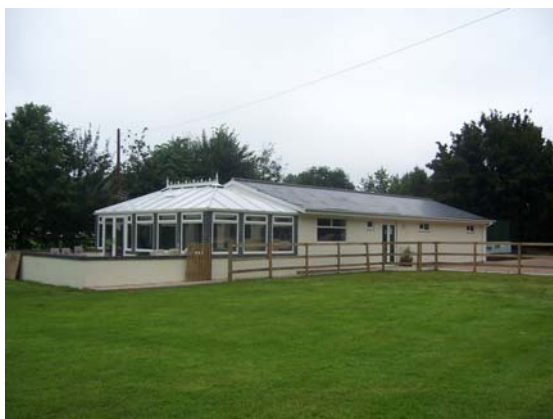
The completed extension, paving and fencing
