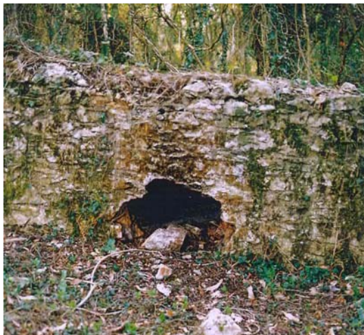
The ancient wall prior to restoration
