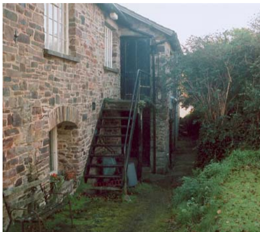
The rear of Georgeham Village Hall prior to the construction of the extension
