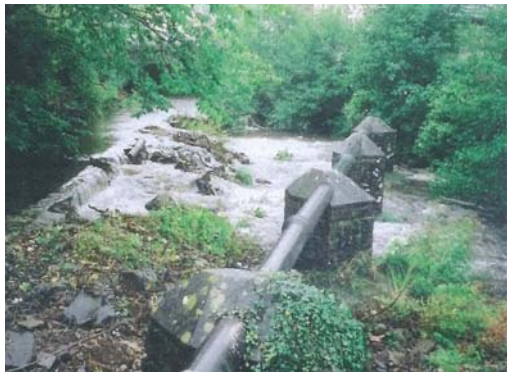
Weir prior to clearance work
