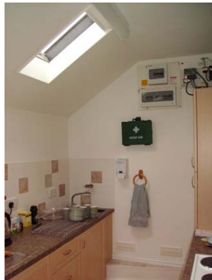
The new kitchen and skylight
