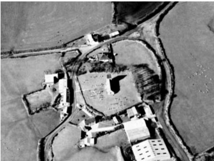
Plate 12: Aerial Aerial photograph of Hollacombe Parish Church, showing its surrounding circular enclosure. (© Devon County Council)
