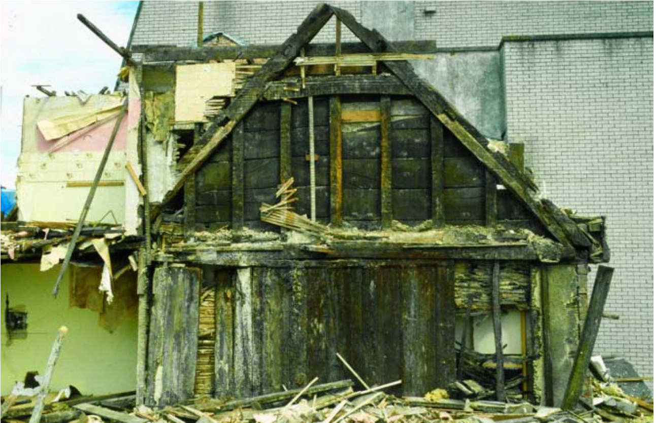
Plate 3: Remains of a 16th century roof and partition incorporated in a later building, and revealed only during demolition for development in Newton Abbot (© Exeter Archaeology)
