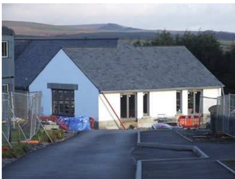
Princetown Village Centre - under construction December 2008
