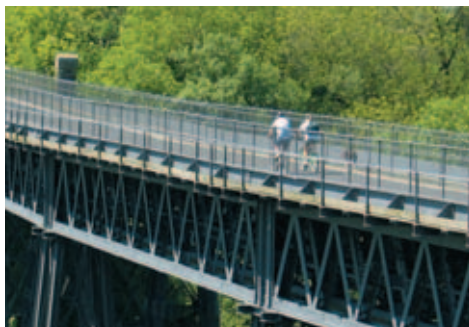
Meldon Viaduct, Granite Way
