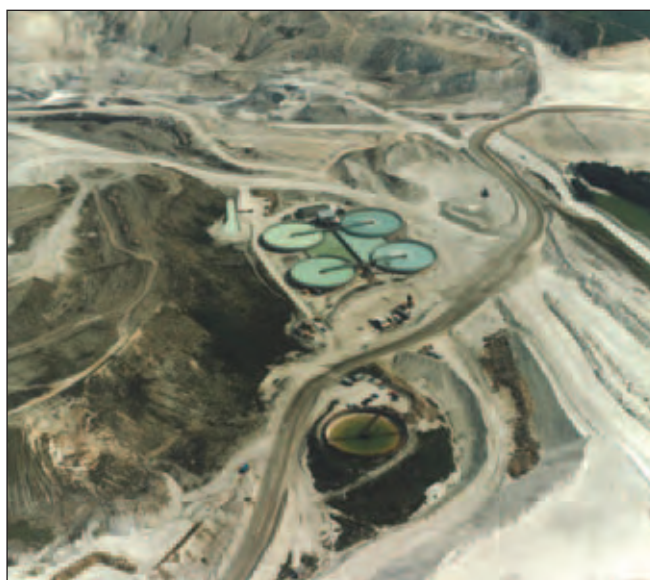
Aerial view of clay thickening plant, near Cholwichtown Pit.
