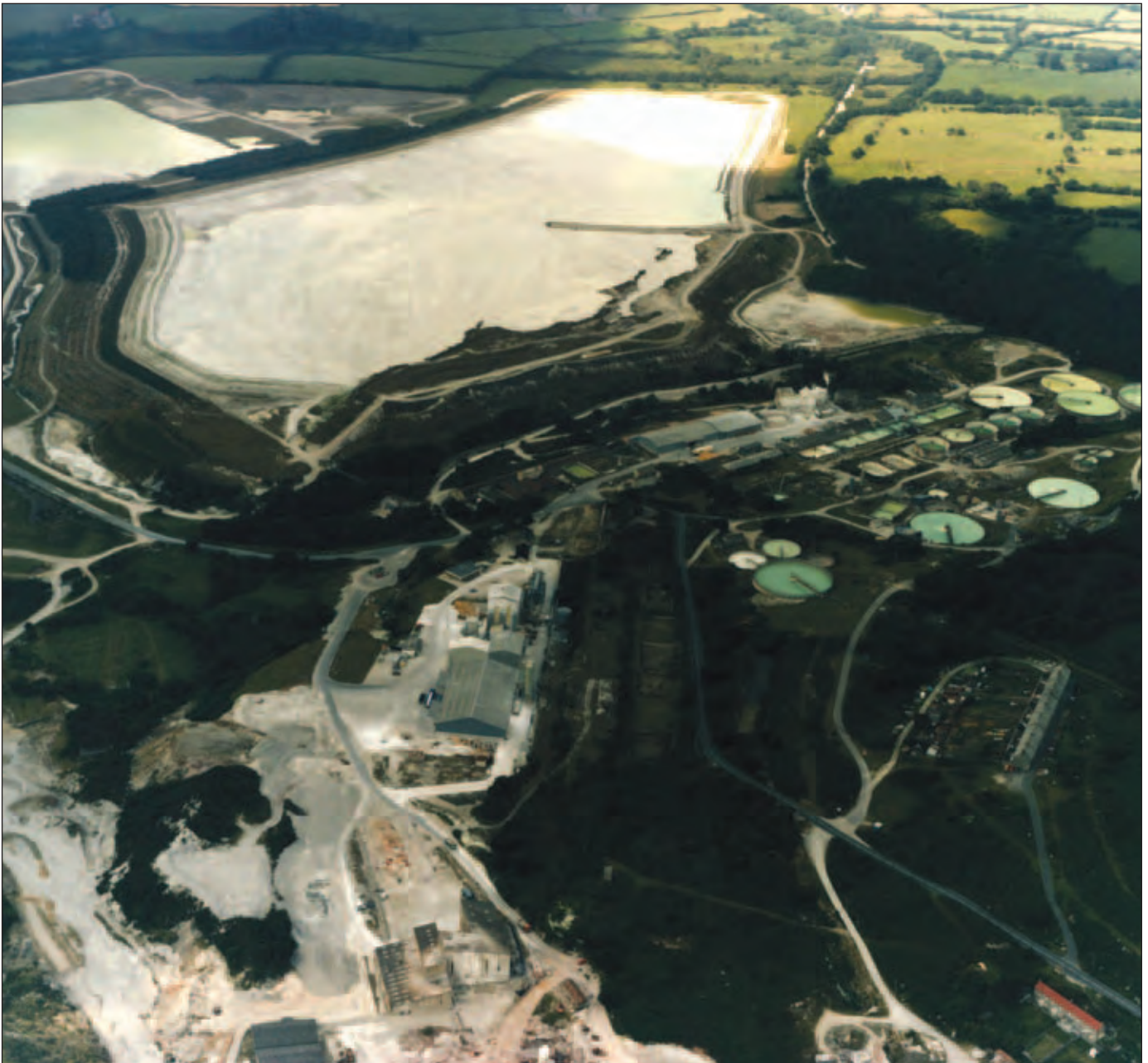
Portworthy processing plant and mica dam.
