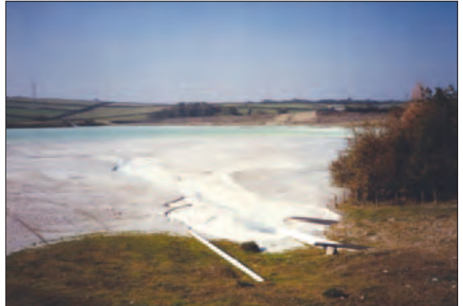
Inflow pipe of the Portworthy Mica Dam.
