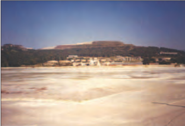
Portworthy Mica Dam with clay thickening plant beyond and tip T2 on the skyline.
