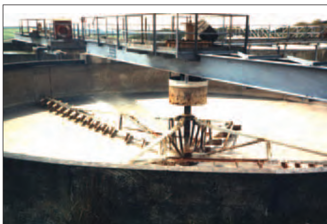
Empty clay thickener undergoing cleaning and maintenance.
