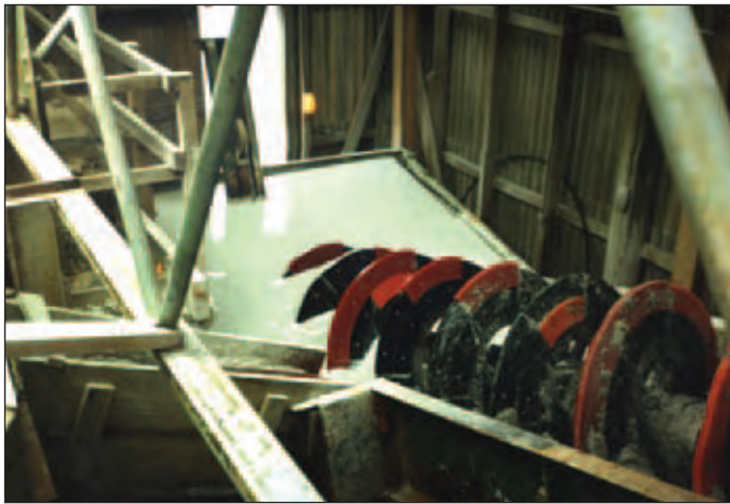
Lifting clay slurry by Archimedes Screw, Marsh Mills Processing Site.
