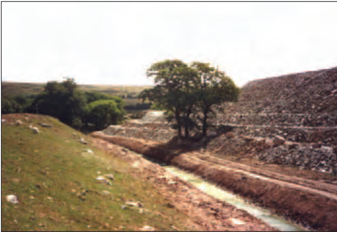
Mica dam retaining wall at Portworthy, Lee Moor
