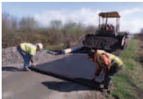
Resurfacing work on The Tarka Trail
