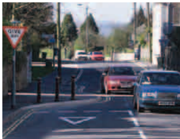
Traffic management scheme at Chudleigh
